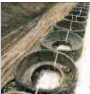
cladding of recycled tyres, plantable and economical
