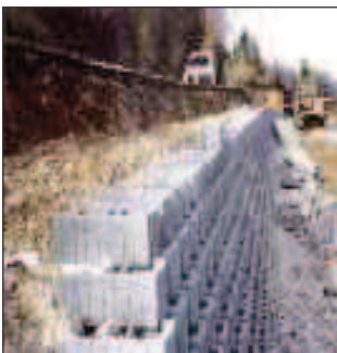
concrete block cladding
