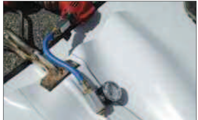
compressed-air weld inspection
